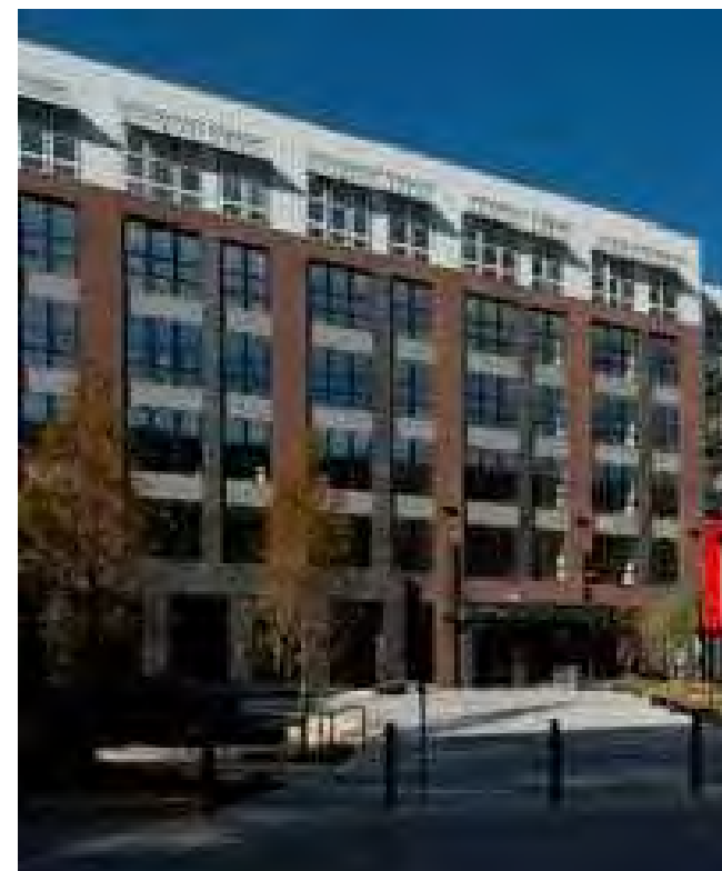
Masonry Fenestration and Brick Articulation
